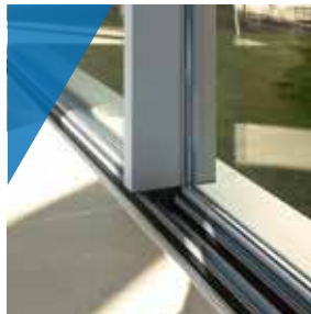
Detail of the central overlap of two panes, showing lower frame flush with the outer and inner pavement.
